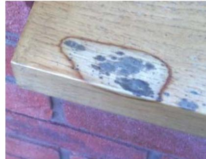
*Staining can be sanded out using a detail sander and the coating system reinstated*
